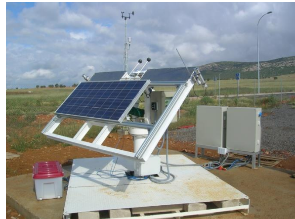
ISFOC Puertollano (SPAIN), 2007
