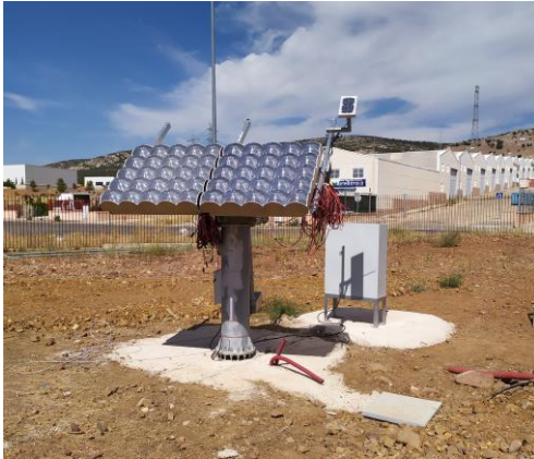
ISFOC Puertollano (SPAIN), 2020
